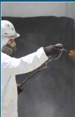
WATCHDOG H3 stays where it's sprayed to maintain consistent coverage of 40 mils cured and deliver hydrostatic head resistance up to 3 times greater than other asphalt-emulsion waterproofing products. WATCHDOG H3 is so reliable, it's backed by a 10-year transferable warranty.\*
