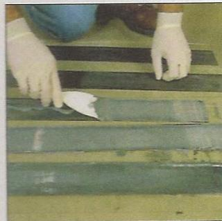
**4. Spread the epoxy** over the plate using a 3/16" v-notched trowel providing a consistent minimum 1/8" thickness.
