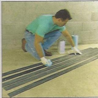
**2. Clean the Reinforcer plates** with an approved solvent. **Do not use a petroleum based solvent.**
