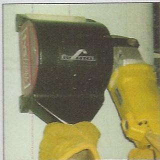
**1. Concrete preparation:** Grind or blast the surface to remove all dirt, paint and uneven surfaces. Then clean the surface.
