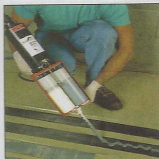
**3. Apply the ECS 104 Structural Epoxy** to the Reinforcer plate.
